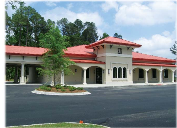
North Office, Valdosta, Lowndes
