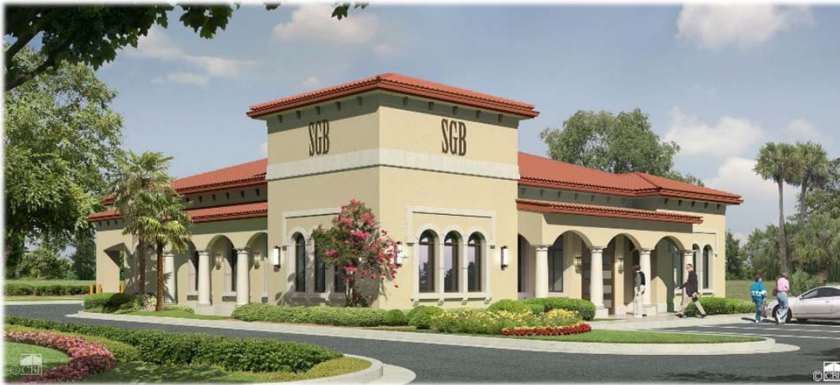
Baytree Office, Valdosta, Lowndes
